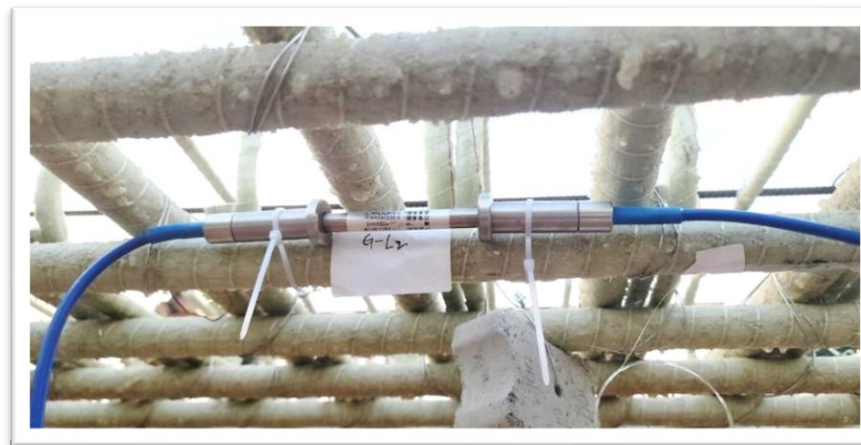
安裝傳感器監測玻璃纖維筋耐久性表現 Sensors installed to monitor the durability of GFRP
